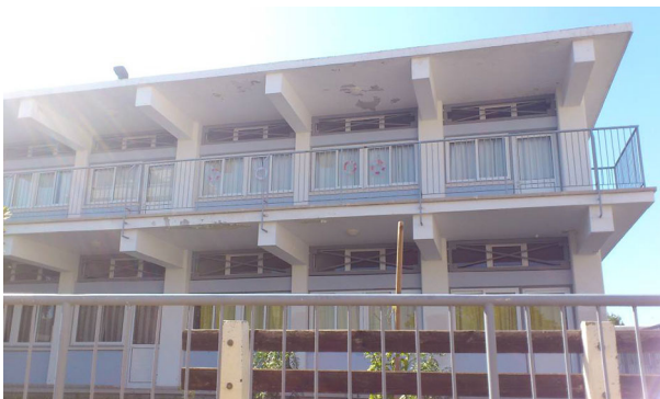
Fig. 1 Front elevation of the R/C school-building
